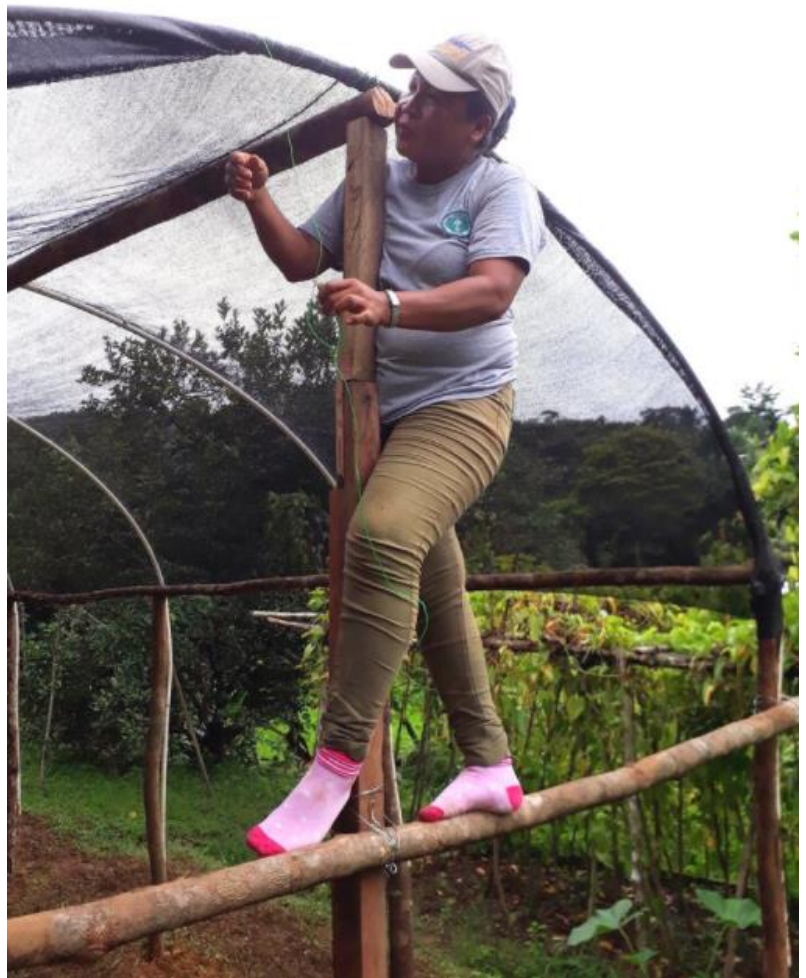
Maribel constructing a hoop house in the community of Aguas Claras in November 2020
